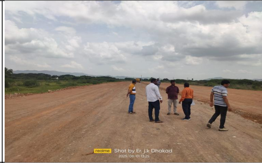
Embankment layer laying work is in progress.
