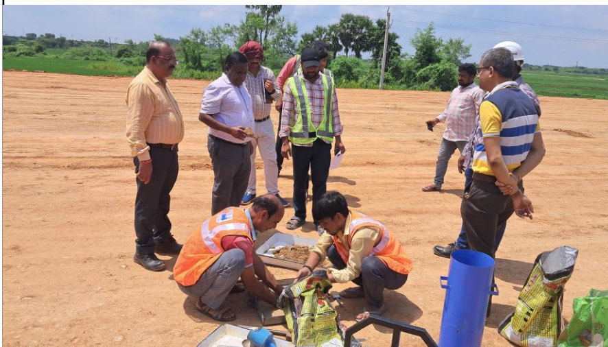
IE's team Site Inspection
