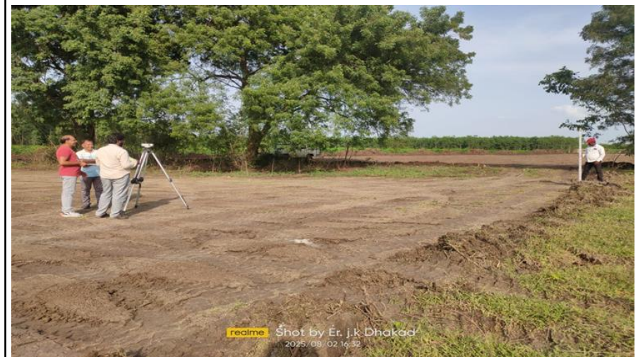
OGL level checking
